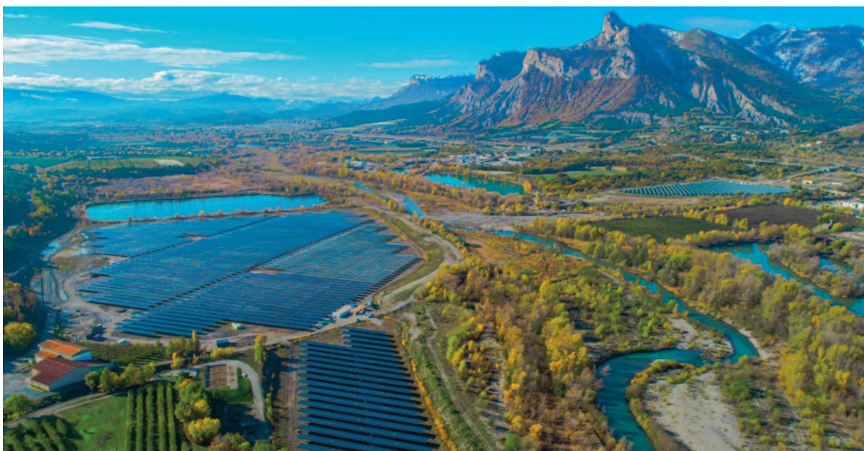
15 MW, Curbans, France.
