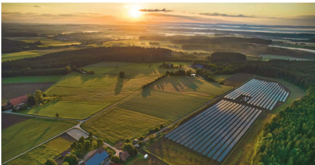
7.27 MW, Pfaffenweiler, Germany.
