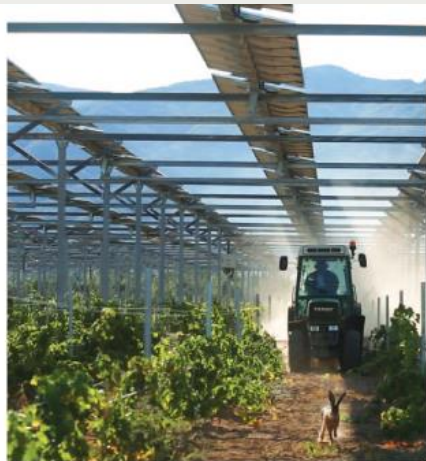
Dynamic shades Agri-PV system, viticulture.
