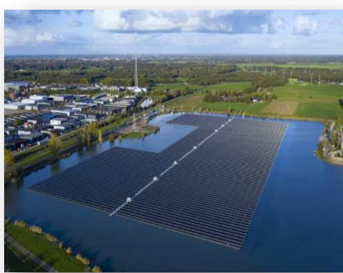
Floating Solar Farms
