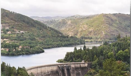
Pumped Hydro Storage
